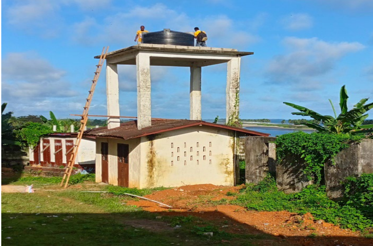
We sponsored a Water System Project to supply water throughout the entire school building.
